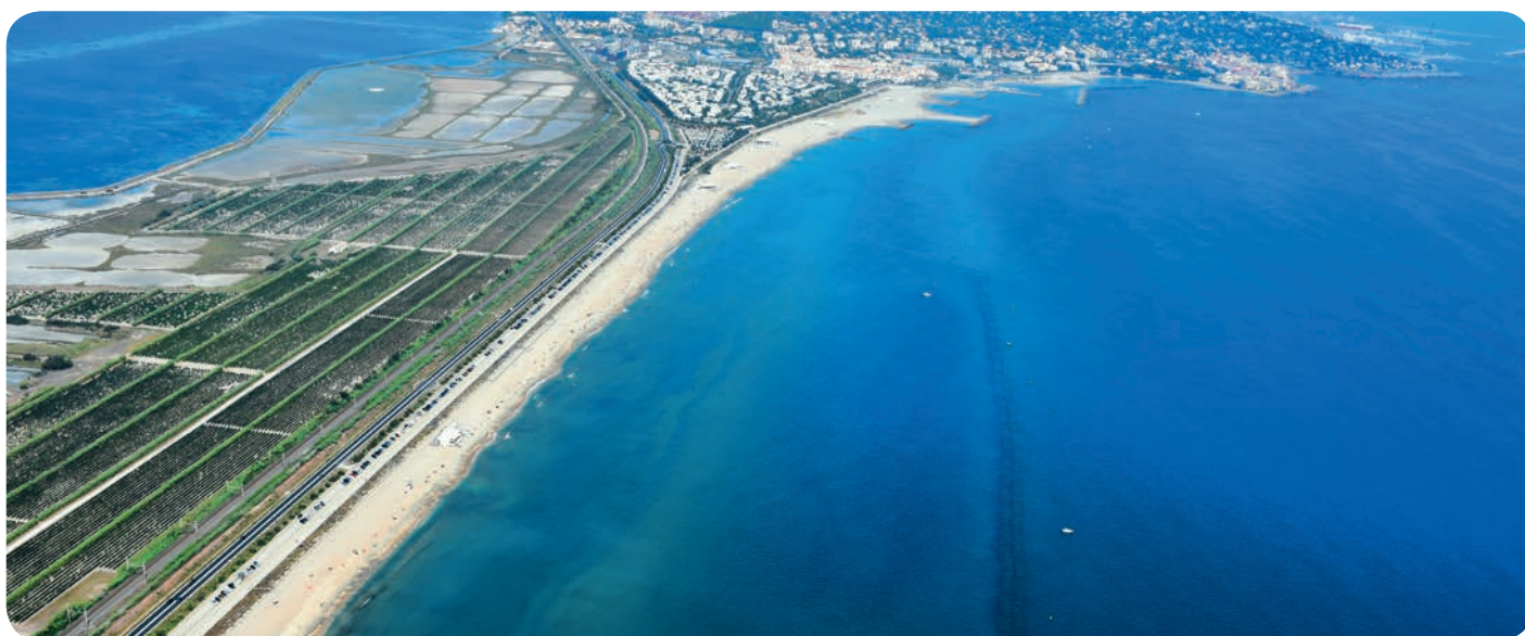
▲ Geotube breakwater for beach protection in Sète (France). © BRL/GL
